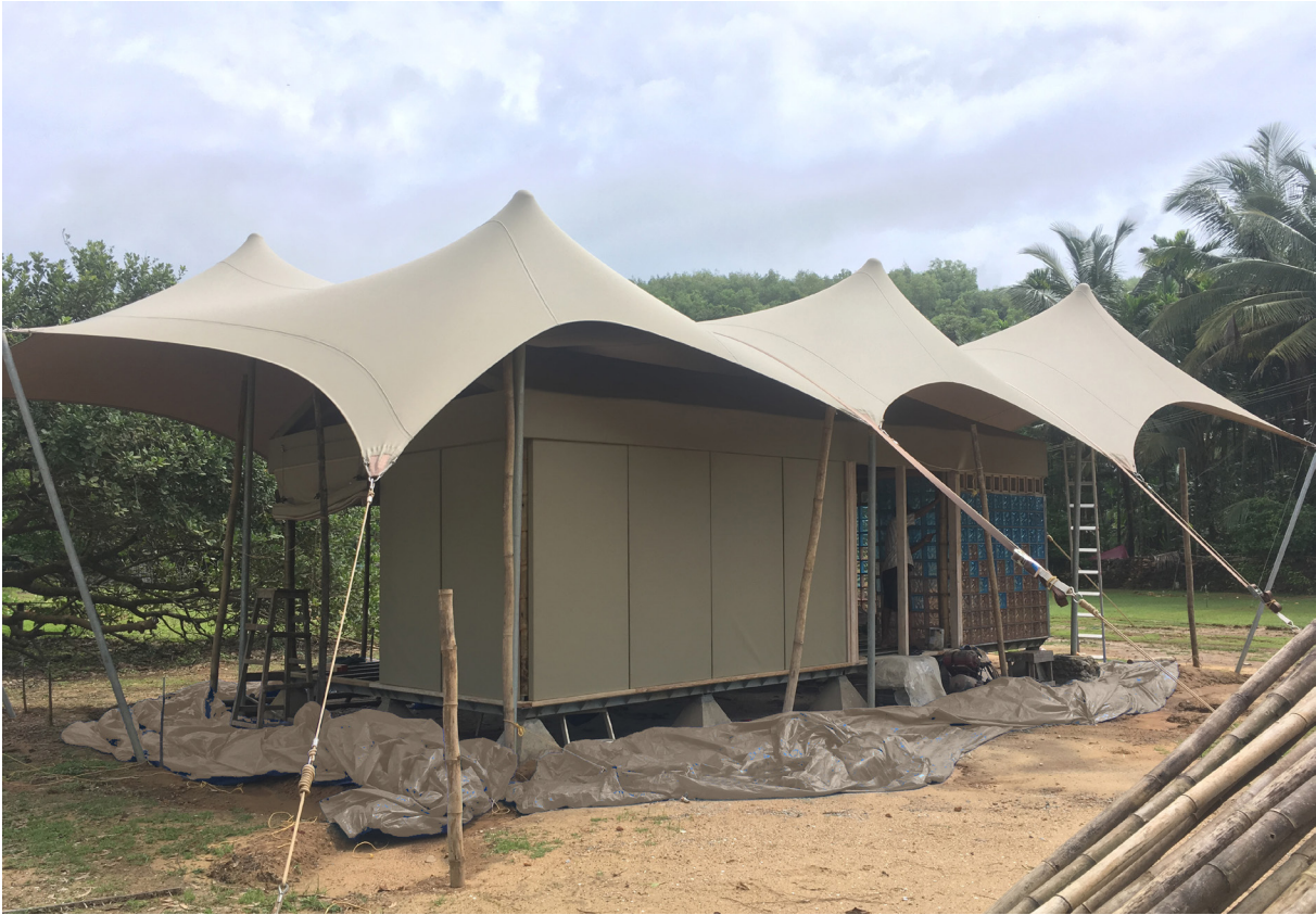
Assembly of wall panels covered in rip-stock fabric in progress
