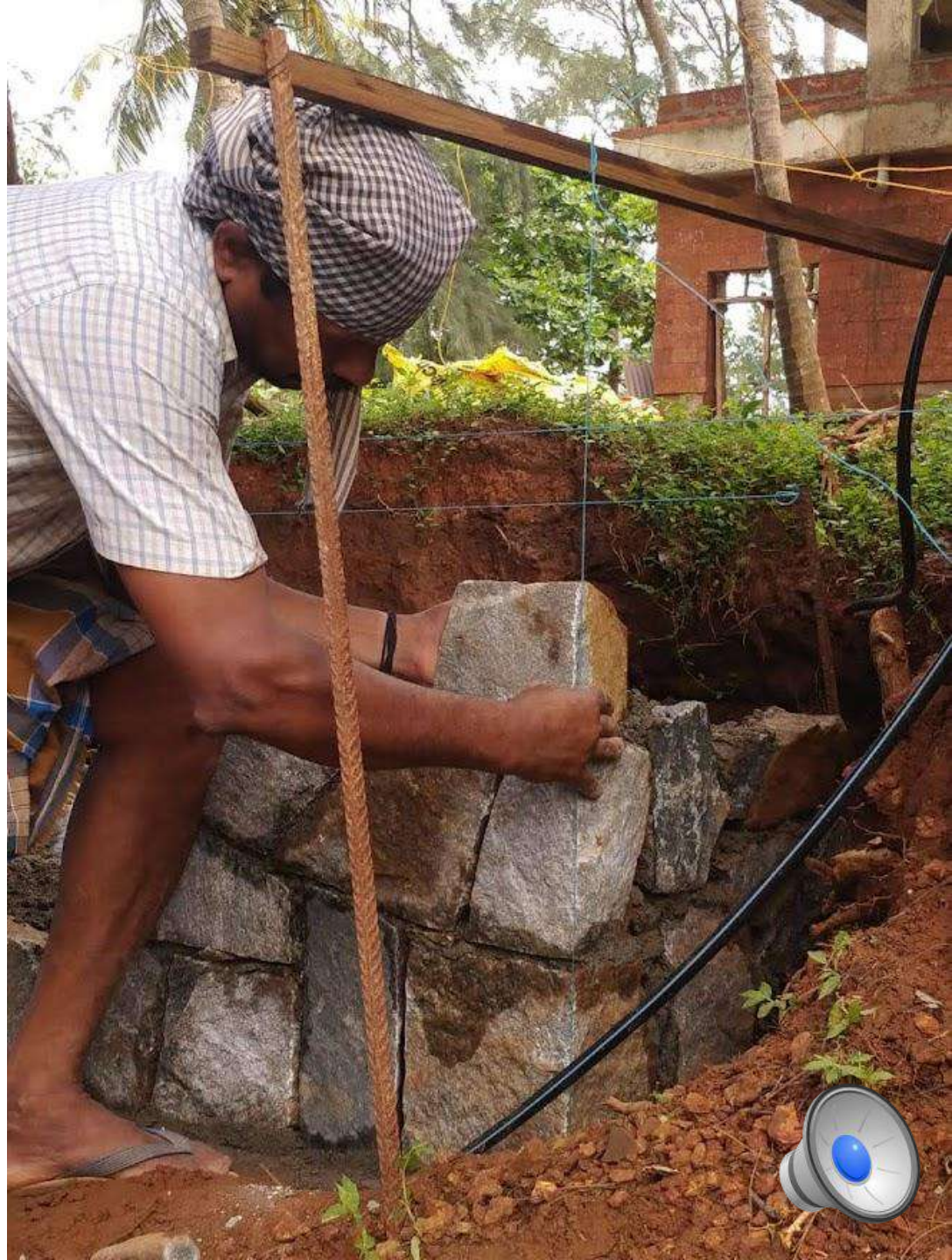
Shile-kallu wall masonry
