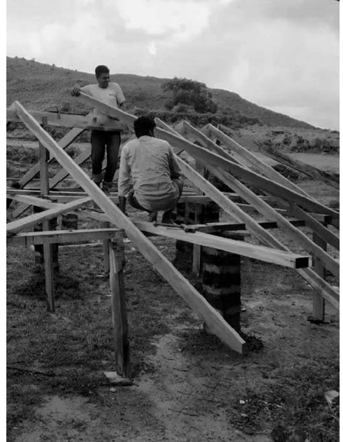
Left : Labeled structural members Above : Off -Site detailing and Assembly
