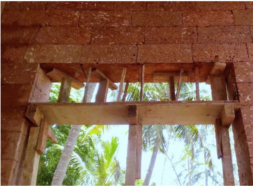
Lintel cladding dressed on-site
