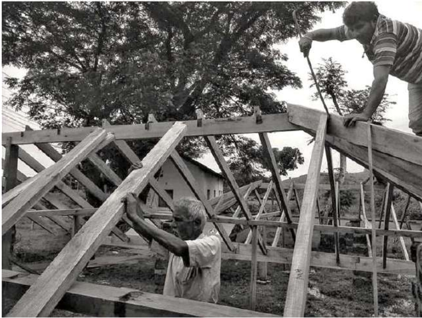
Off - Site Assembly
