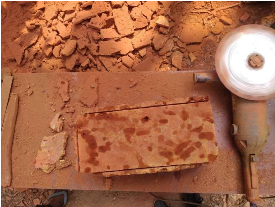
Processes : Papercut laterite dressing, On-site, Kirubeli Cove Retreat and Wellness Centre
