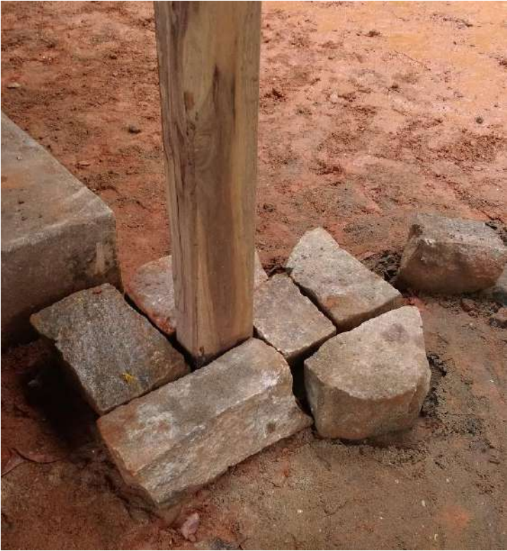
Above : Shile-kallu Paving Right : Shile-kallu Splitting
