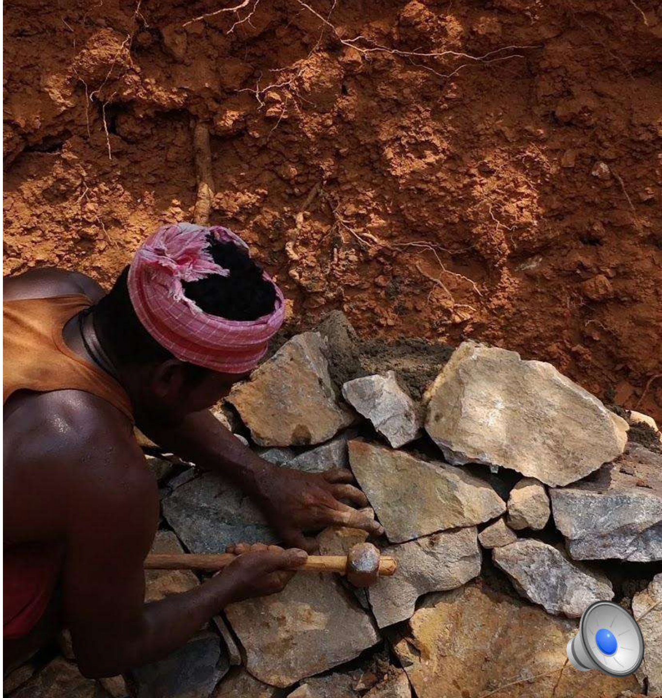
1:1 mock-up of retaining wall : dry stone masonry
