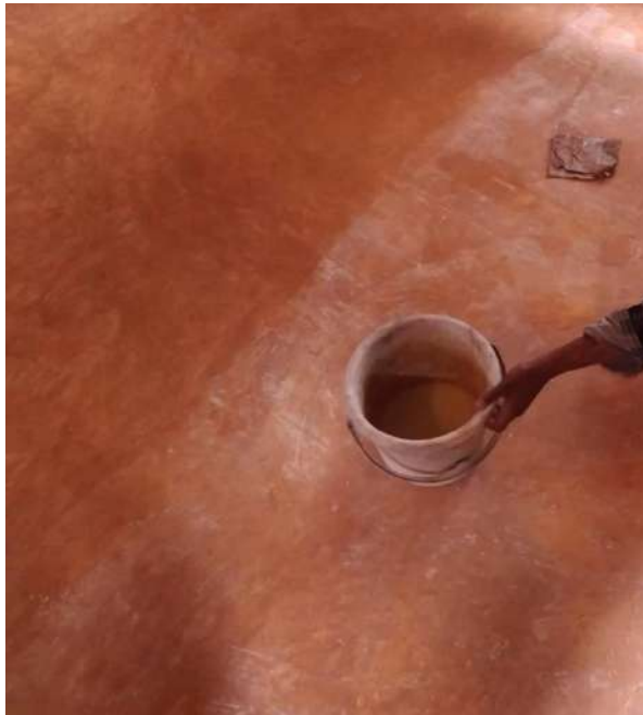
Above : Applying Wax polish on oxide floor Right : Scrapping of dried wax layer.
