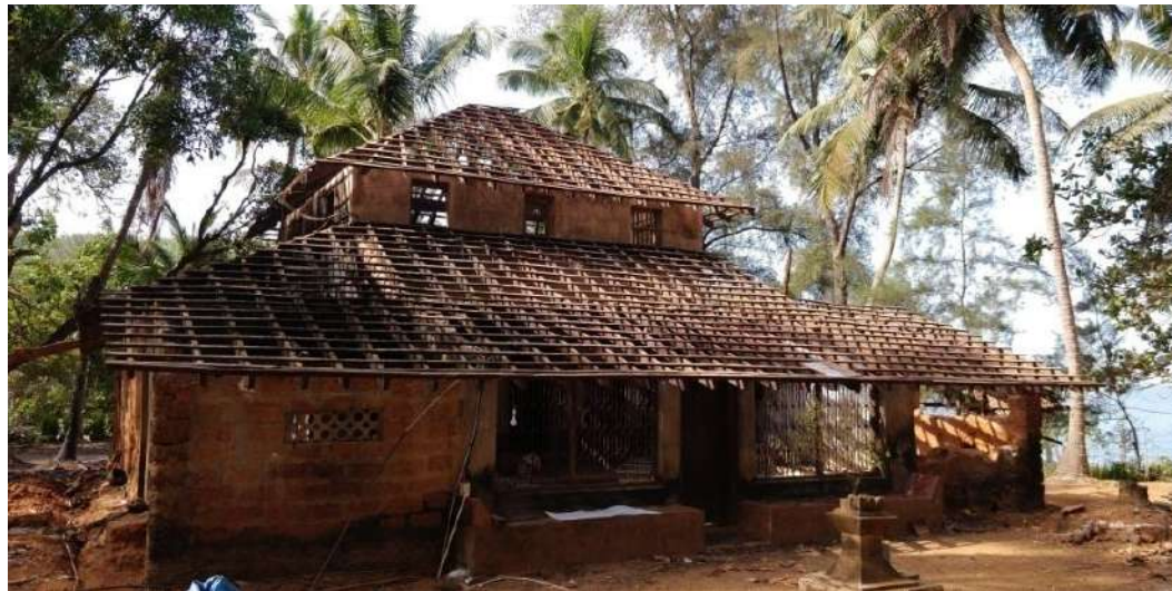
Deconstruction of the Existing house, Kirubeli Cove
