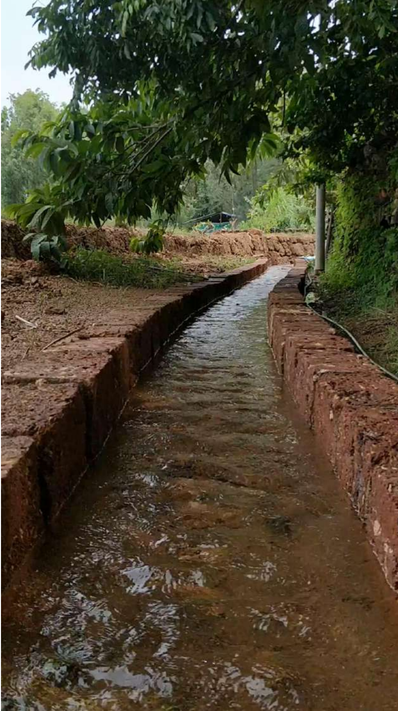
Left : Storm water runoff drain Right : Sweet water well
