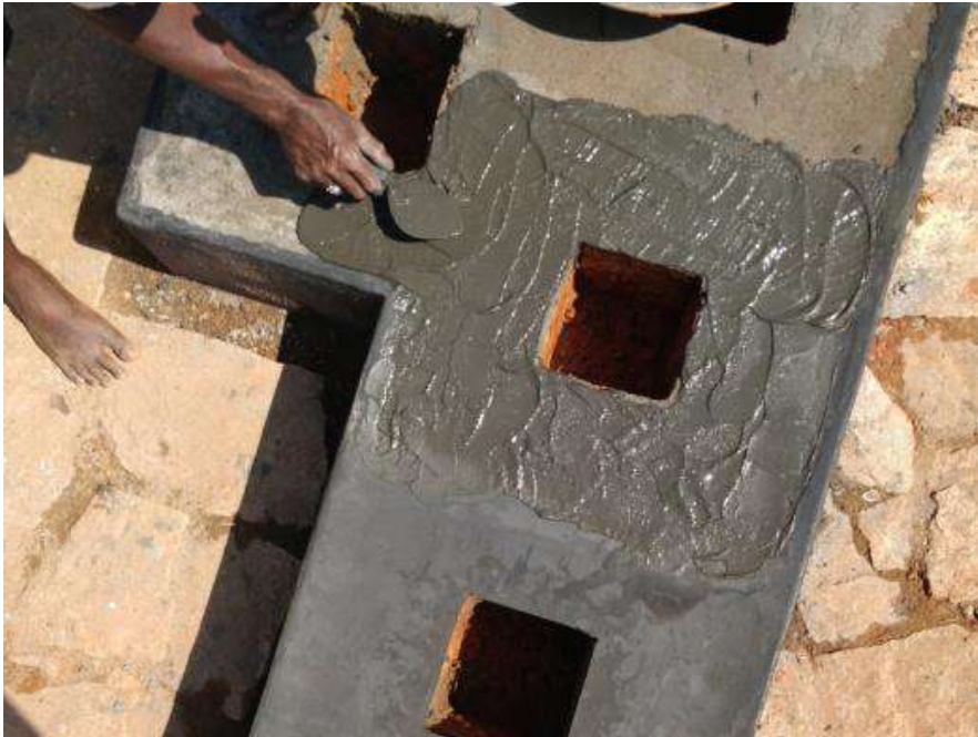
Above: Applying Slurry- like oxide mixture Right Top : Curing of oxide with rice husk Right Bottom : Scrubbing with coconut coir
