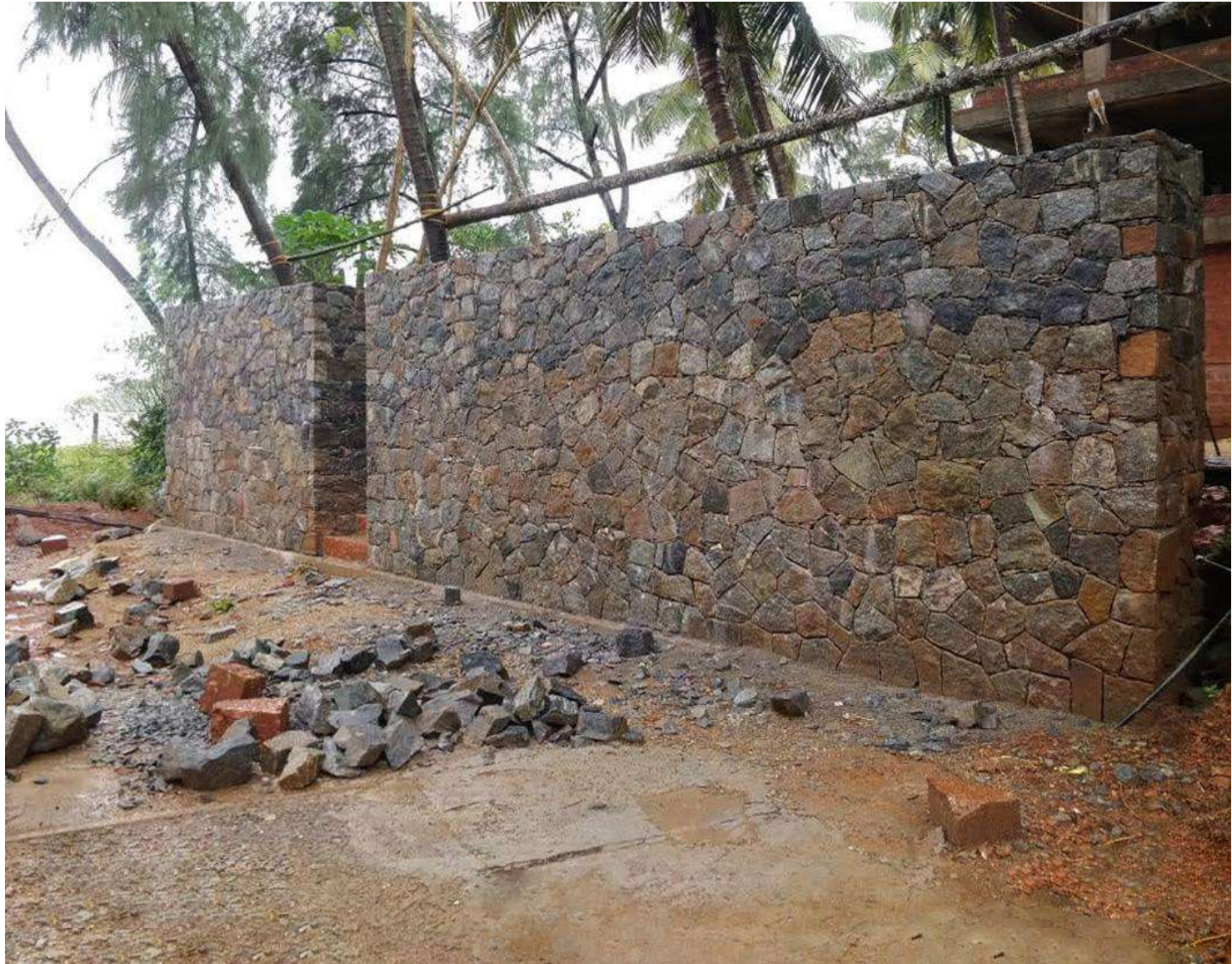
Shile-Kallu Wall Masonry, Outdoor Showers
