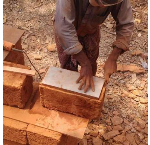
Processes : Papercut laterite dressing, On-site, Kirubeli Cove Retreat and Wellness Centre
