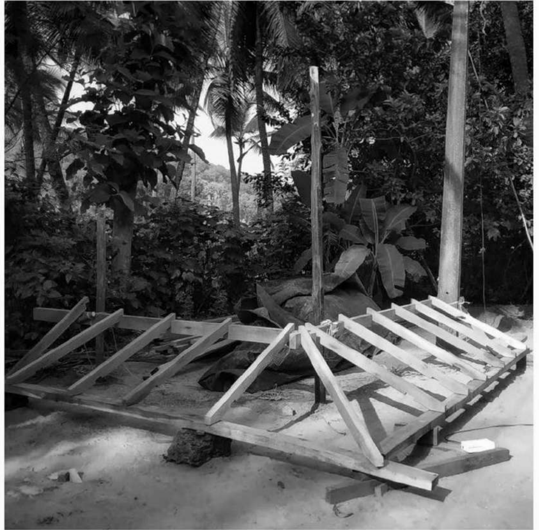
Off Site Detailing and Assembly
