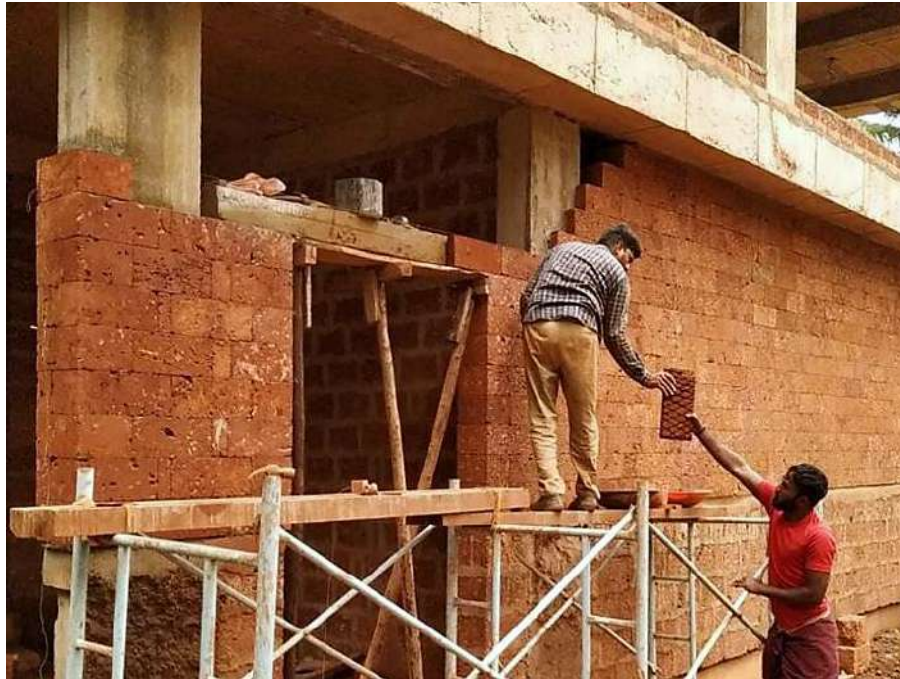
Papercut Laterite Masonry in progress, North wall, Core Structure
